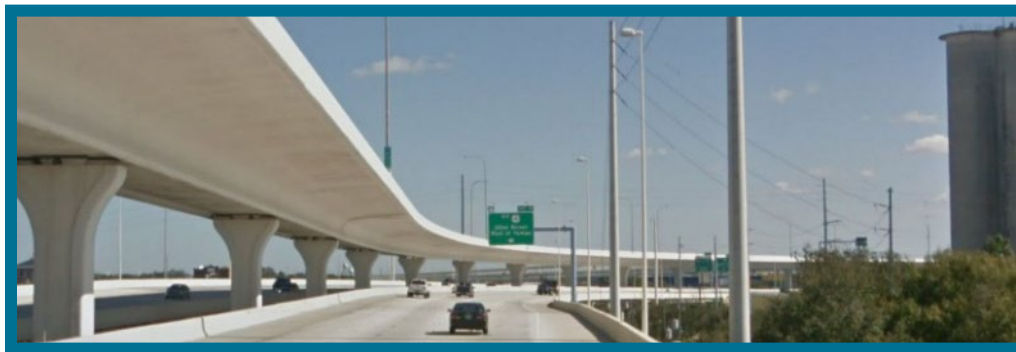
Exhibit 9. Elevated reversible lanes on the Lee Roy Selmon Expressway.
