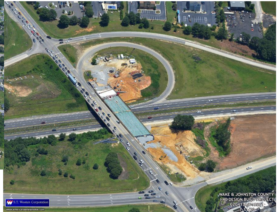
Shift traffic to temporary pattern on NC 42 late Fall 2020
